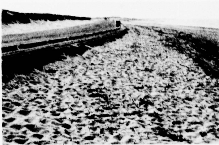
Photo 1. January 1967. The effect of sand fences in dune building is easily seen in this aesthetic view of southern Nauset Beach, Chatham. The now removed Old Harbor Coast Guard Station looms in background.
