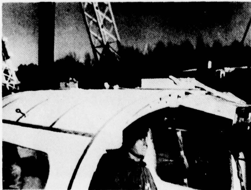
Figure 2-8. - Post-crash condition of substructure, partial of roof
