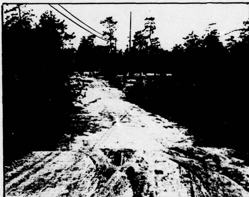
Auxillary spillway near right abutment
