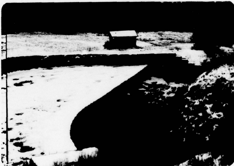
Paved spillway apron leading to rock gorge.
