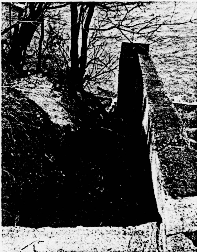
Erosion behind left wingwall structure
