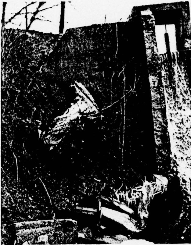
Deterioration of right wingwall structure
