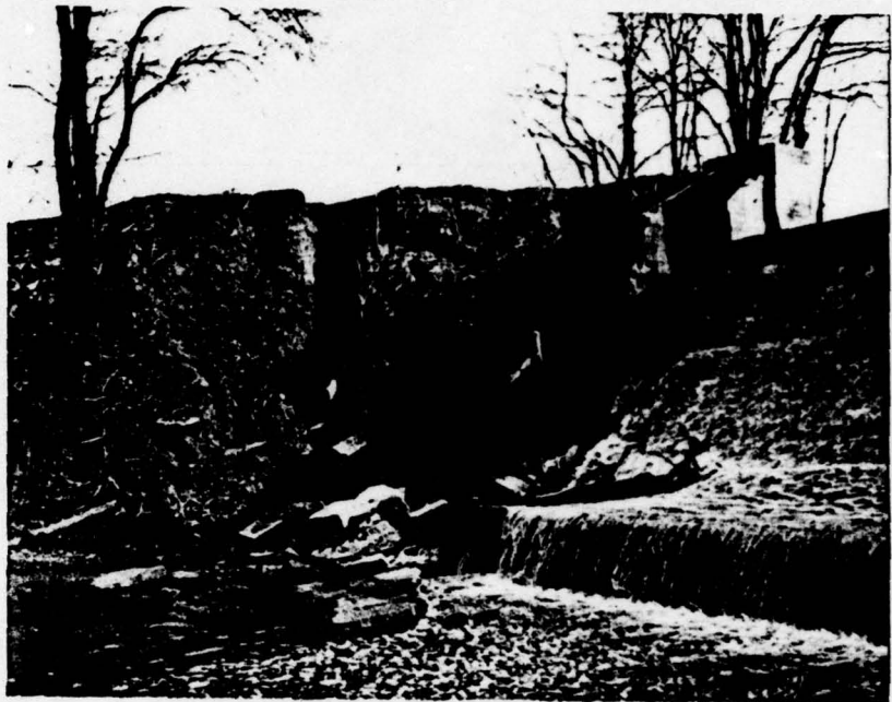
Erosion of right embankment
