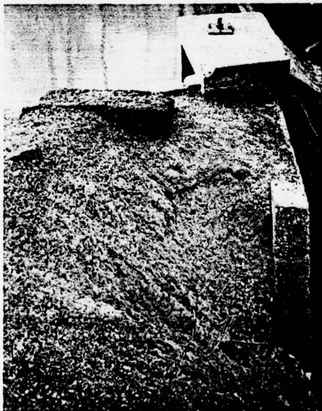
Sloughing and structural cracking at right wingwall
