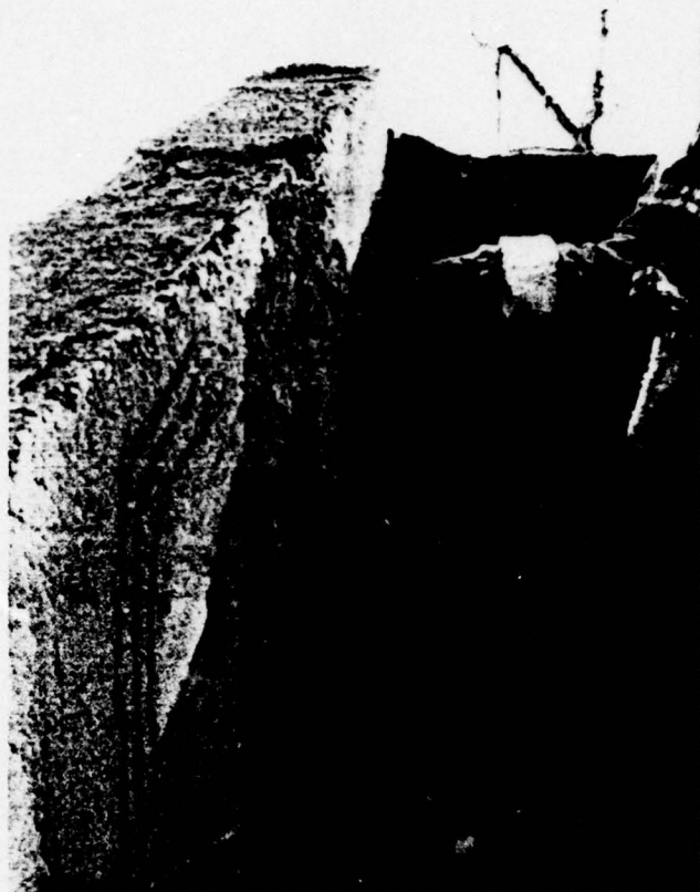
Structural cracking at juncture of left wingwall and abutment
