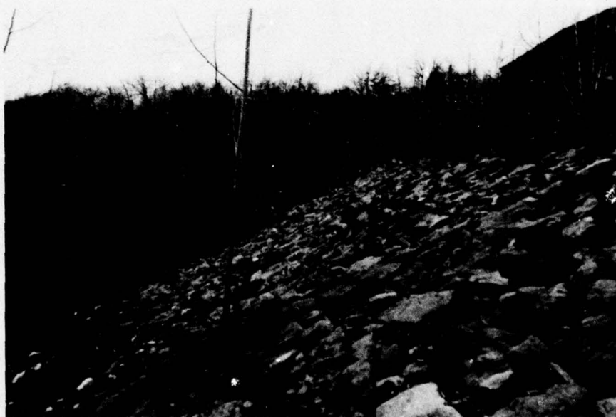
Photo 2 - Hand-placed rock facing above the downstream embankment bench. (12-2-78)
