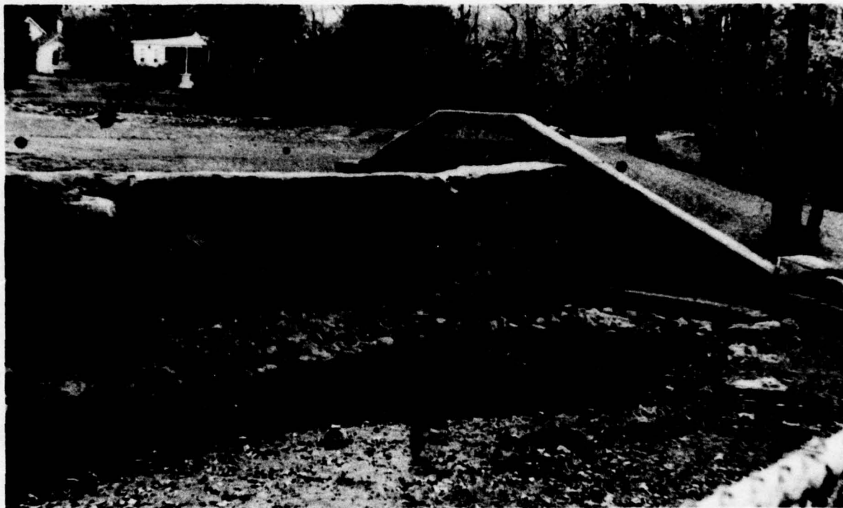
Photo A View of southern half of spillway (Oct. 28, 1973) (Photo courtesy of Haefeli Engineering, P.A.)
