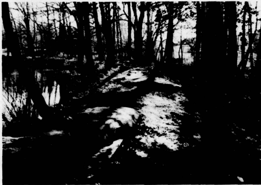
Photo 3 View of embankment crest looking south from spillway
