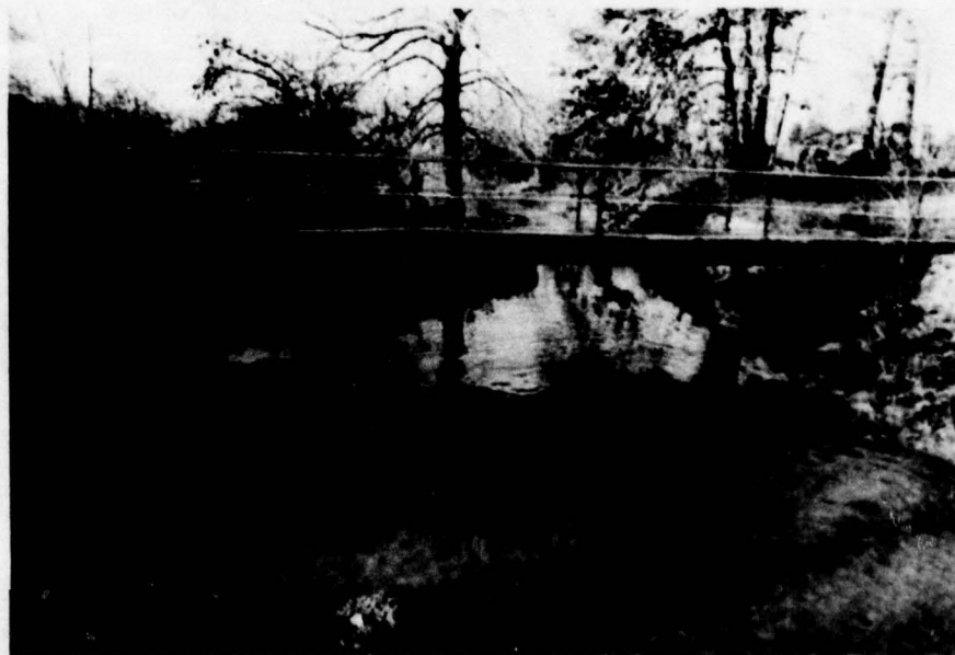
Photo 11 View looking downstream from spillway crest
