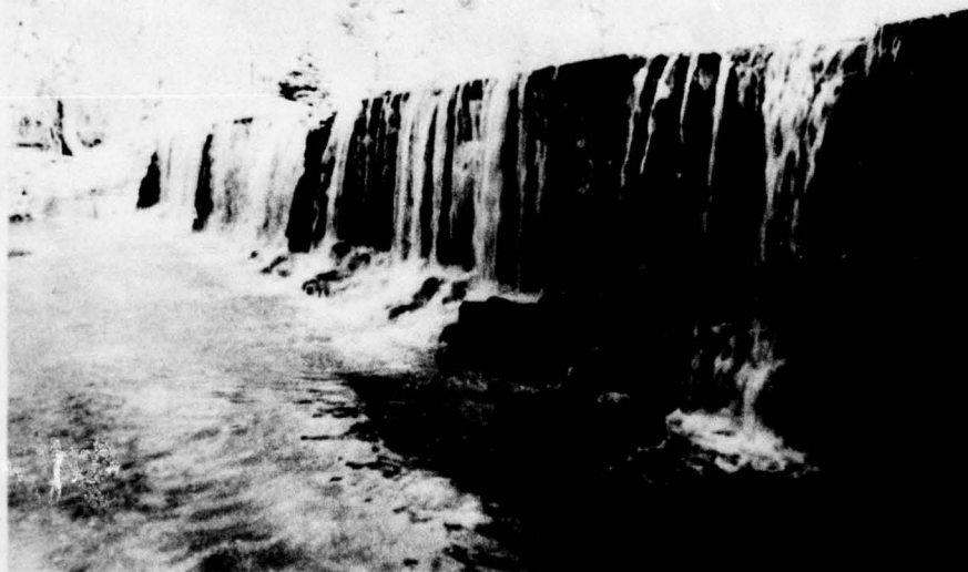
Photo 6 View of downstream face of spillway looking north
