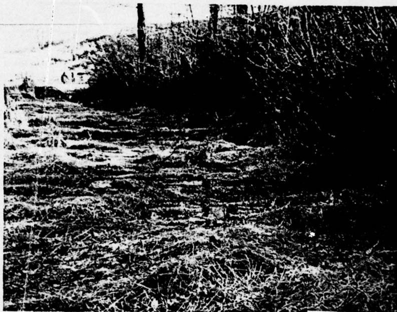
Seepage at toe of left embankment
