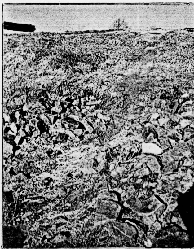
Displaced riprap directly opposite intake structure
