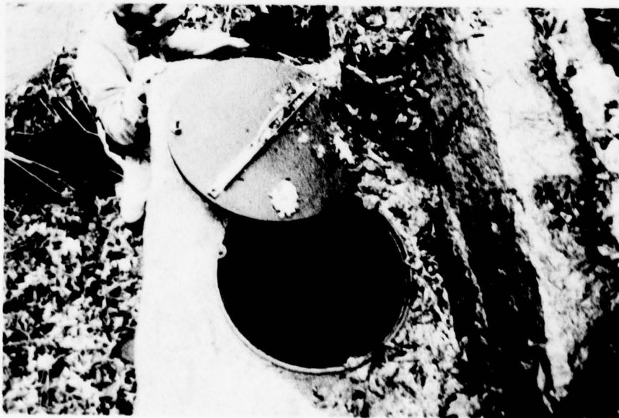
Photo 6 - Valve chamber for 6-inch outlet on left side of dam. (December 4, 1978)
