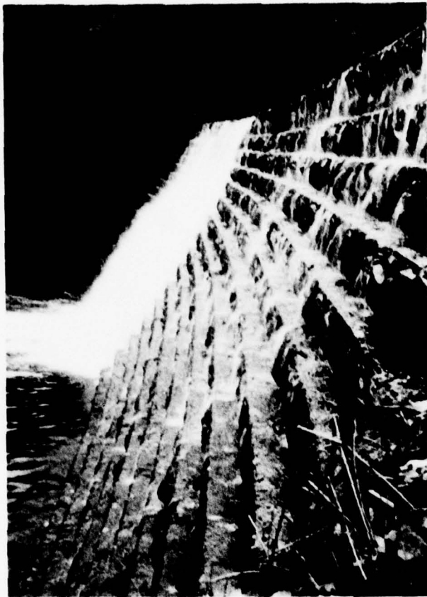
Photo 1 - Downstream face of dam looking west. (December 4, 1978)
