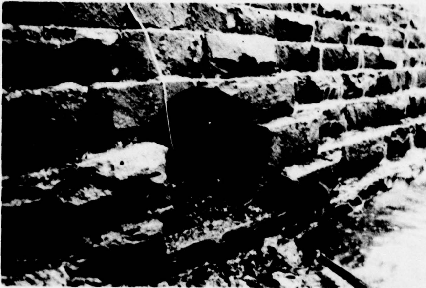
Photo 7 - 48-inch emergency outlet on right side of dam. (December 4, 1978)
