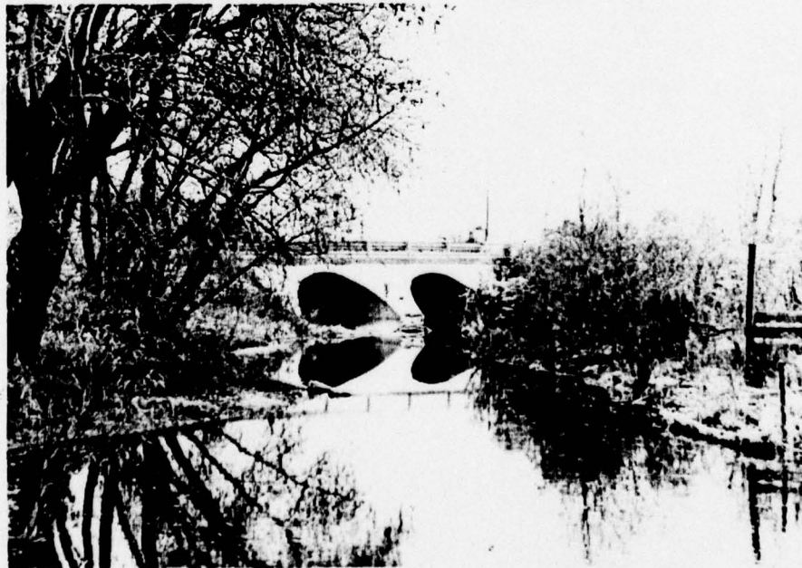
PHOTO 16 View of Route 195 Culverts From Mill Race Channel
