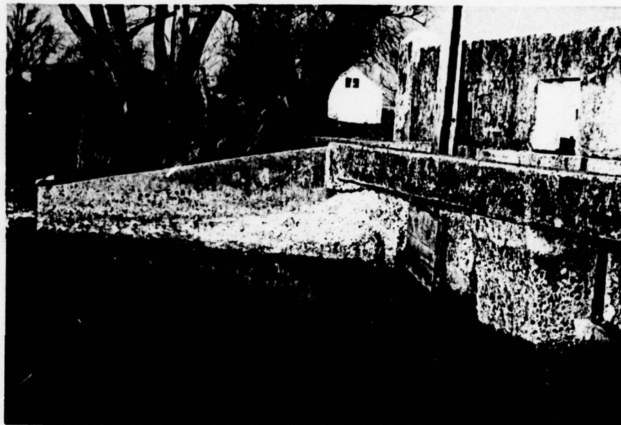
PHOTO 3 Mill Road Dam
