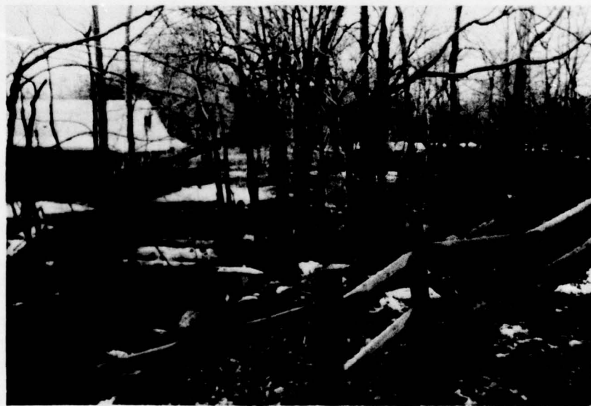
Photo 9 - House on right side of lined channel downstream of spillway. (November 30, 1978)
