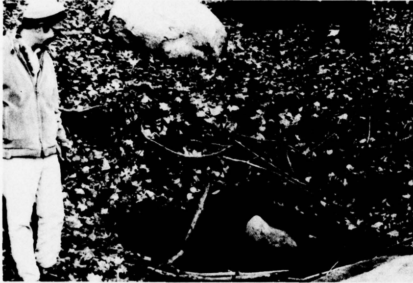
Photo 6 - Reservoir drain outlet obstructed by debris. (November 30, 1978)
