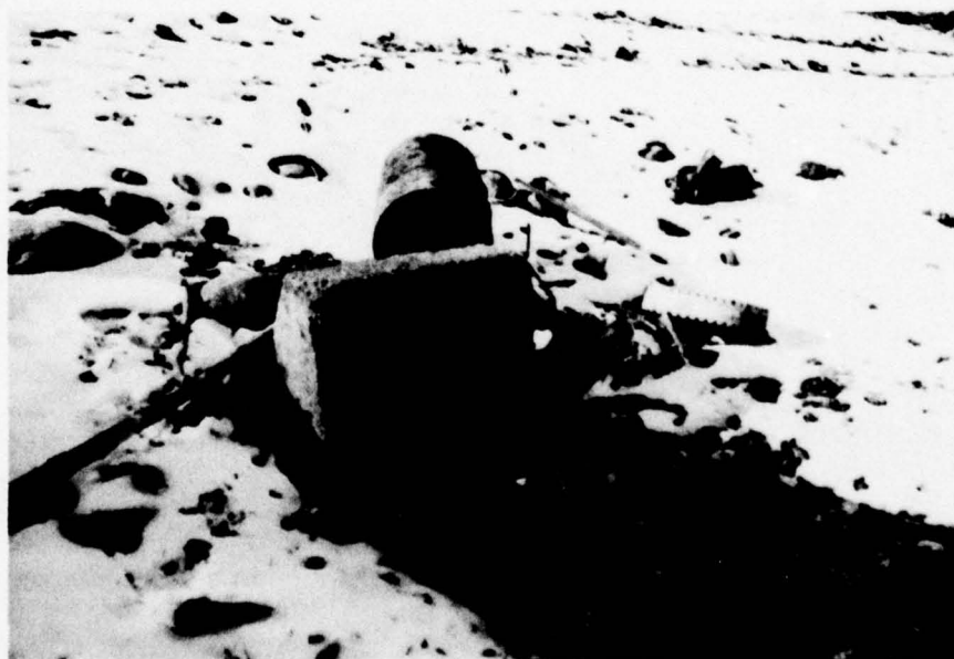
Photo 8 View of intake to outlet pipe
