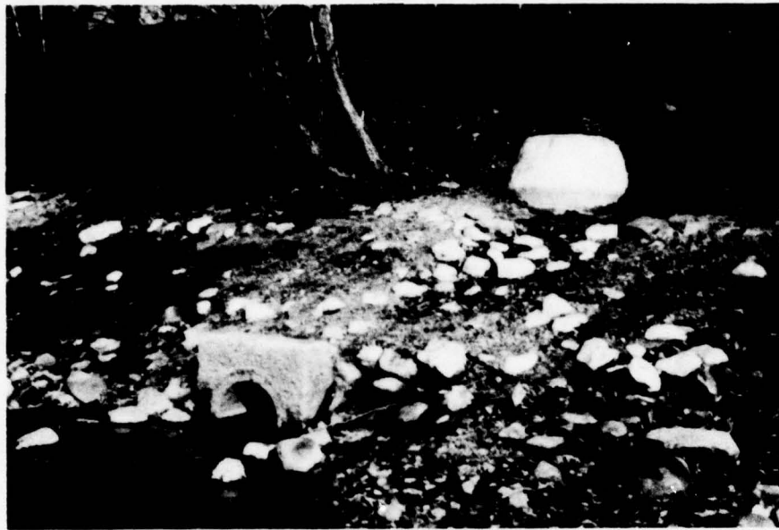
Photo 9 View of outlet pipe and valve chamber at downstream toe of dam
