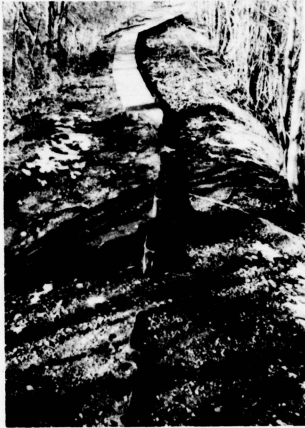
Photo 1 View of embankment crest looking west from spillway
