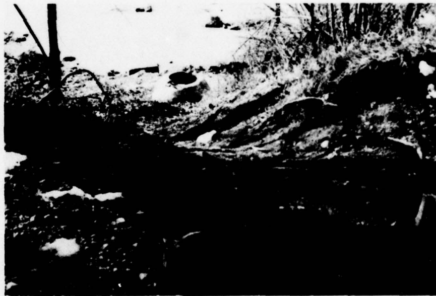
Photo 4 View of gully at eastern end of the downstream face of embankment looking down from dam crest
