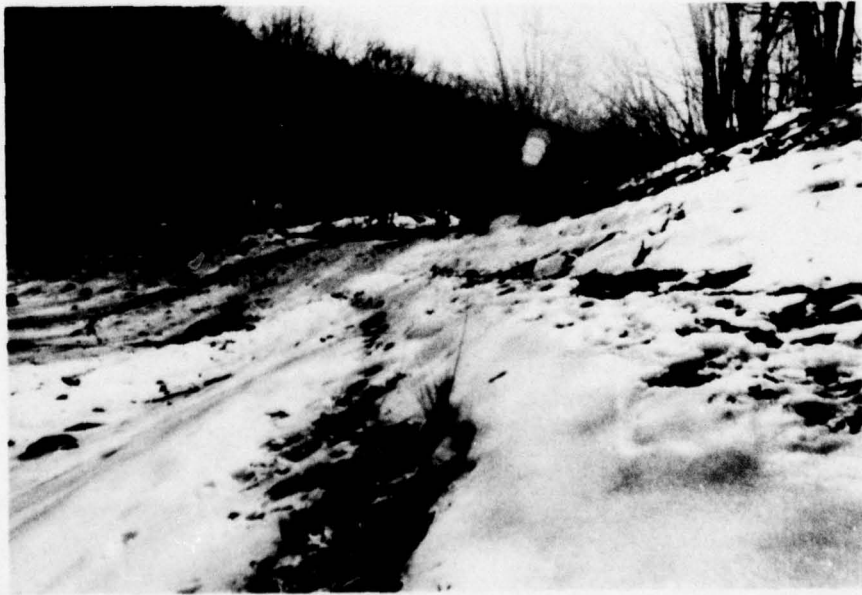
Photo 2 View of upstream face of dam looking east
