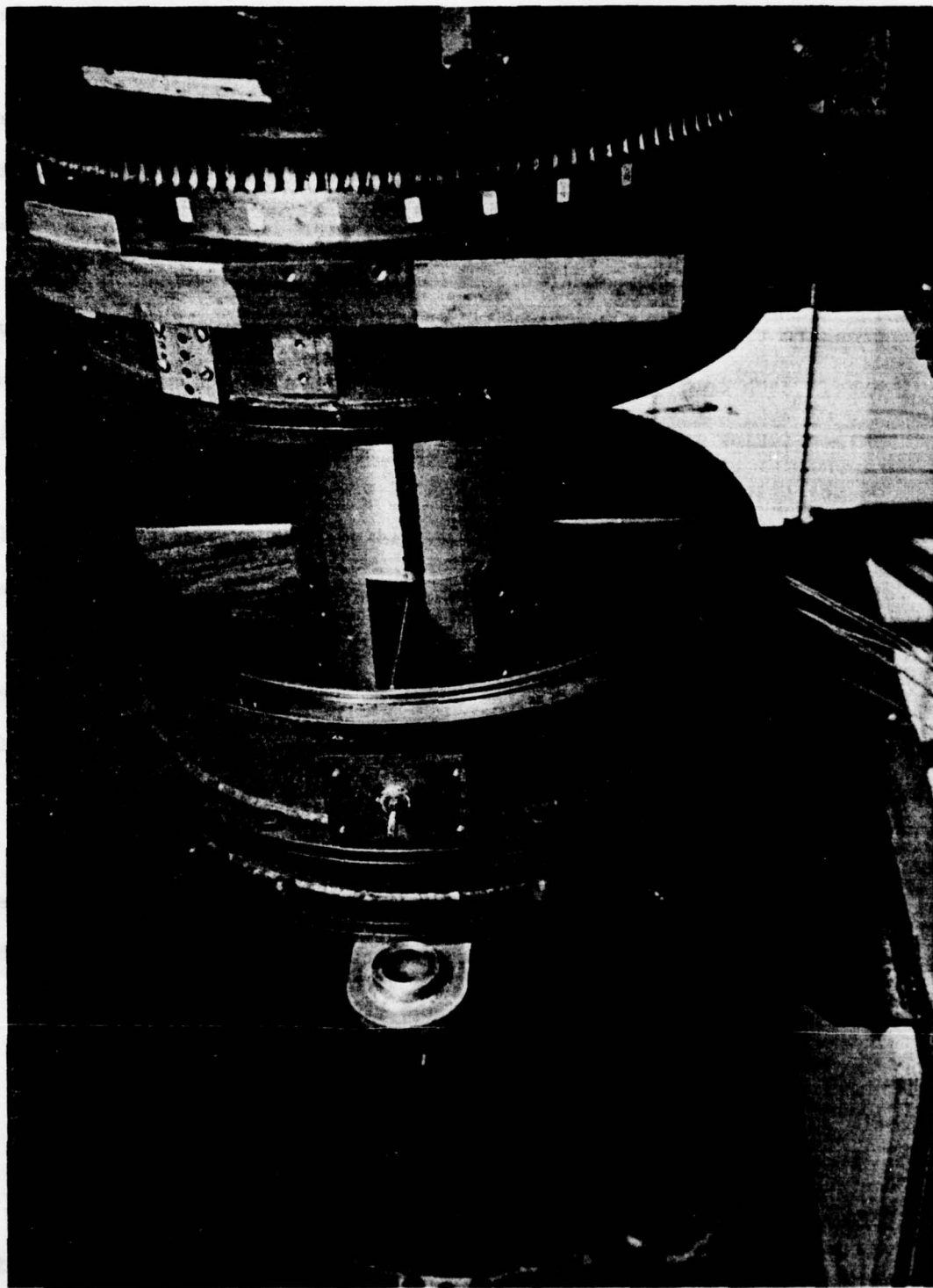
Figure 11. Installation of Stators in AFRR
