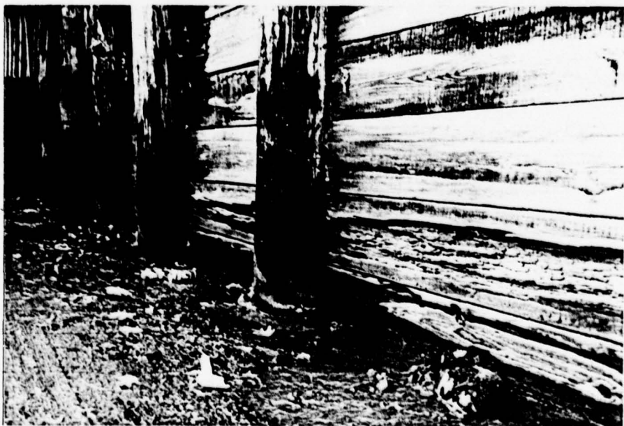
Rotted timber planking in spillway structure
