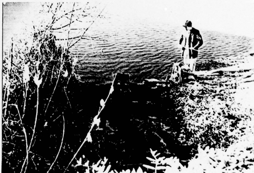
Auxillary spillway to old mill race
