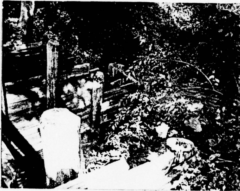
Spillway outlet structure
