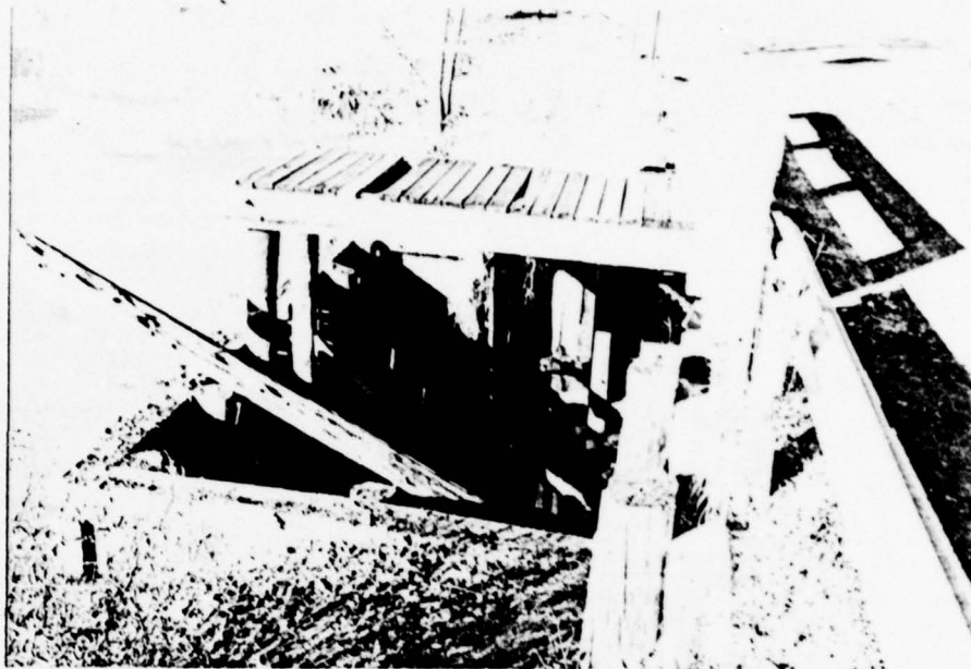
Timber box spillway
