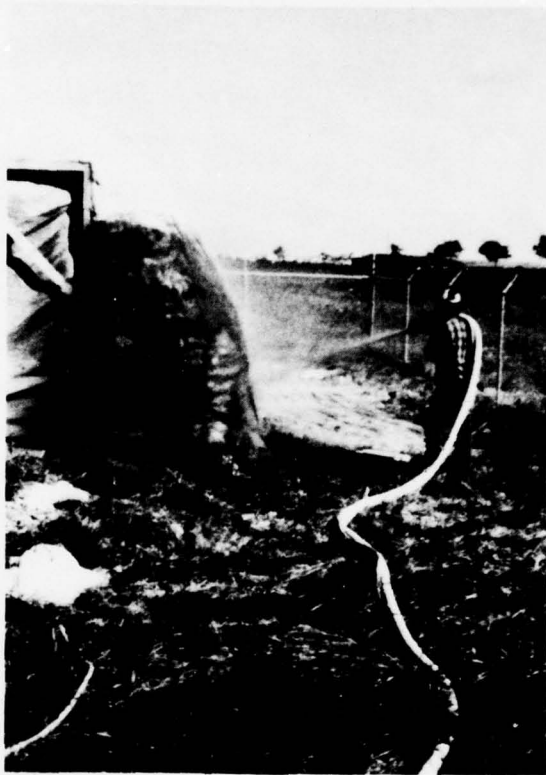
Figure 9. Application of shotcrete.
