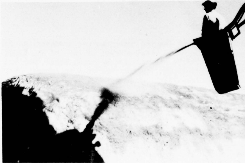
Figure 11. Shotcreting from bucket crane.
