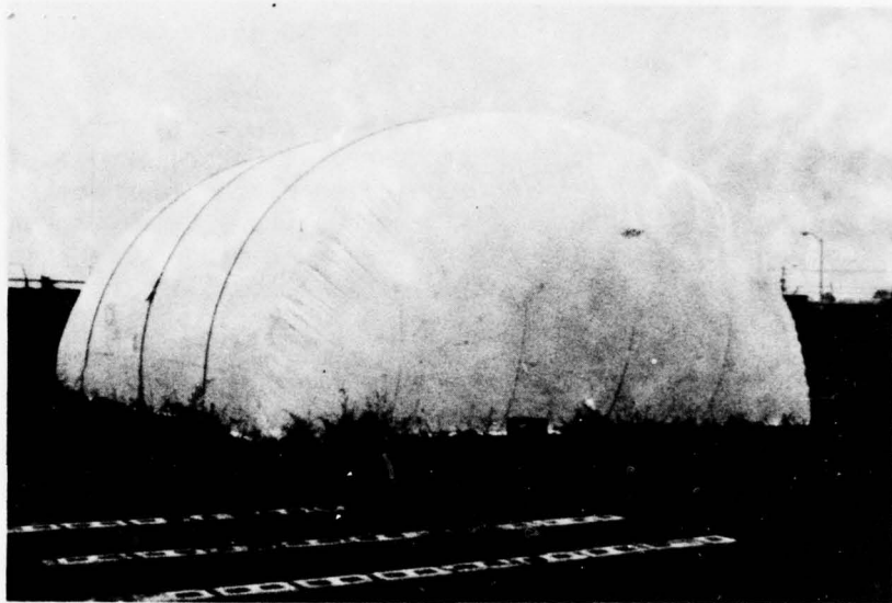
Figure 6. Inflatable form showing safety ropes.
