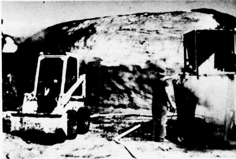
Figure 10. Hopper positioned above shotcrete machine.
