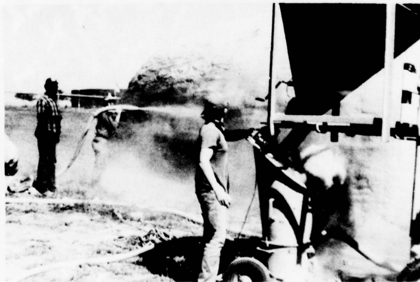
Figure 13. National Guardsman spraying shotcrete.
