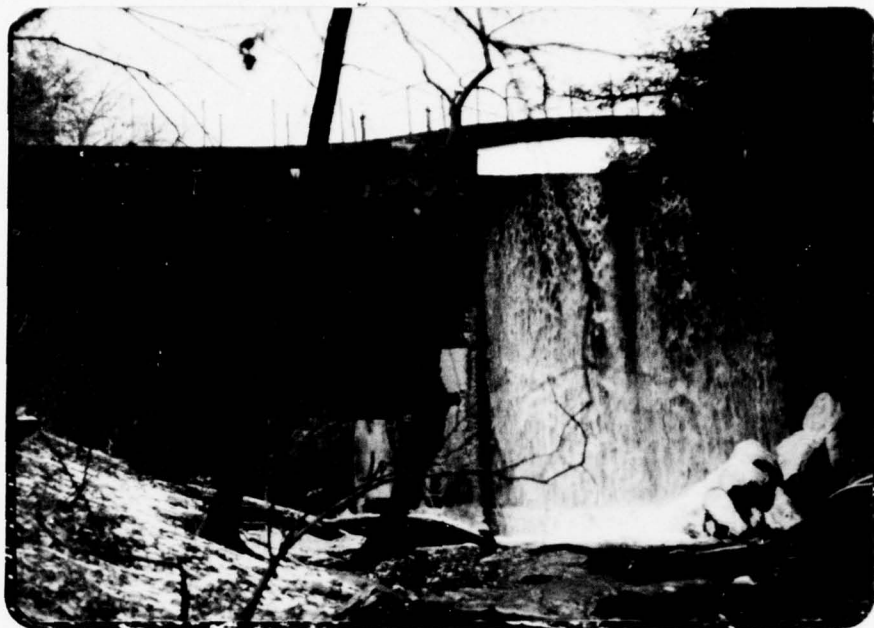
Downstream right face of dam and spillway. Looking upstream.
