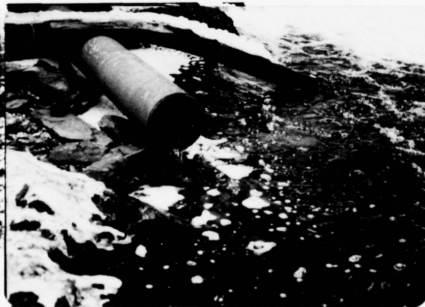
12-in-dia outlet pipe. Outlet pipe is below tail water.
