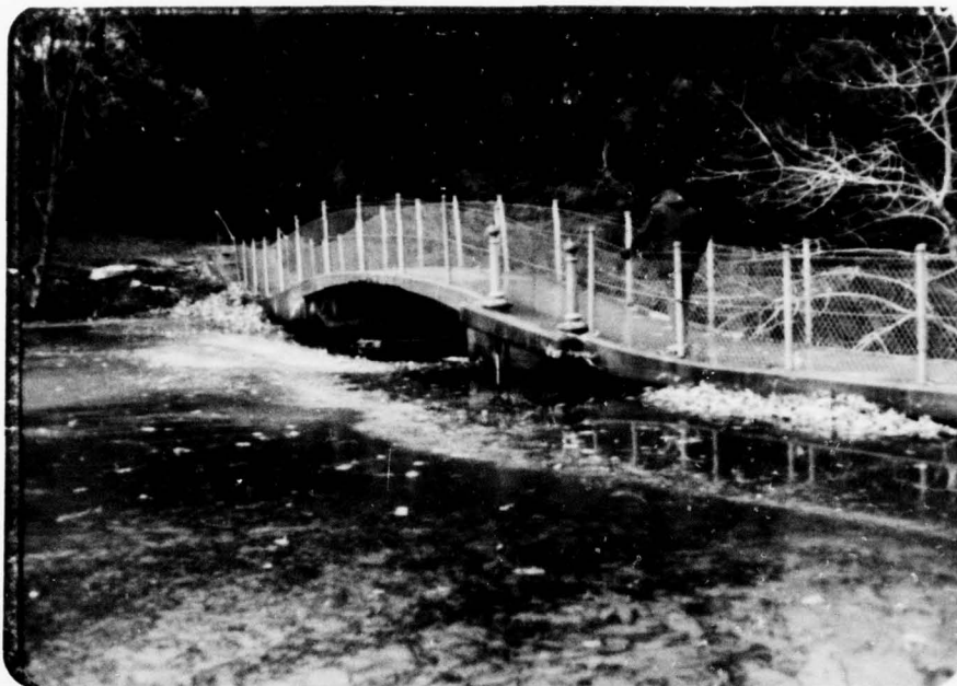
View of upstream crest of dam and gate valve operators. 21 December 1978
