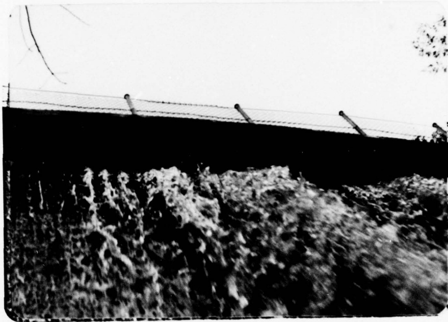
Spillway crest below foot bridge.
