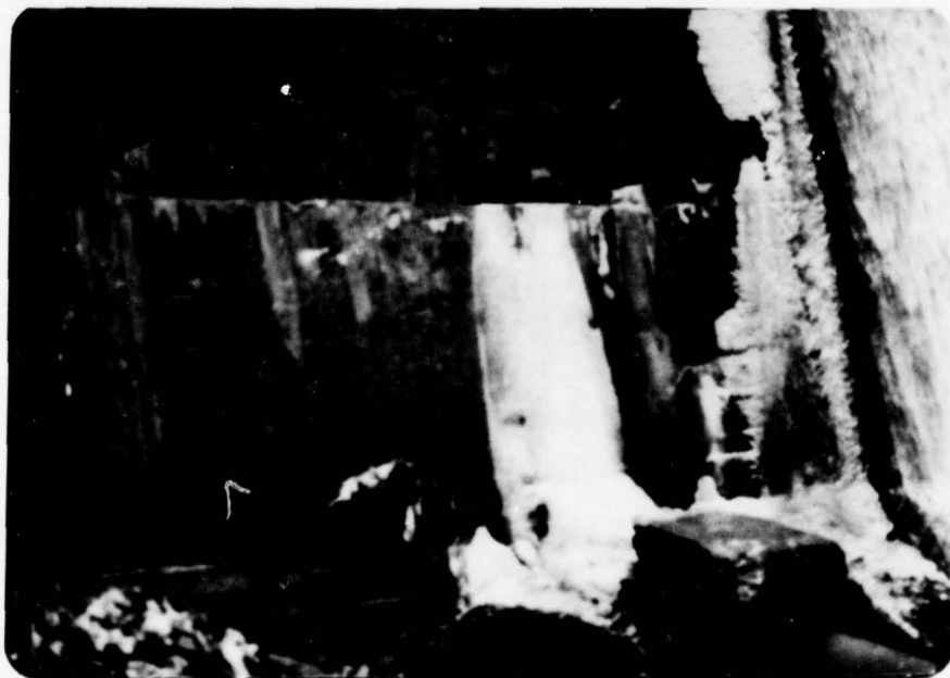
Leakage through dam at right side of spillway.
