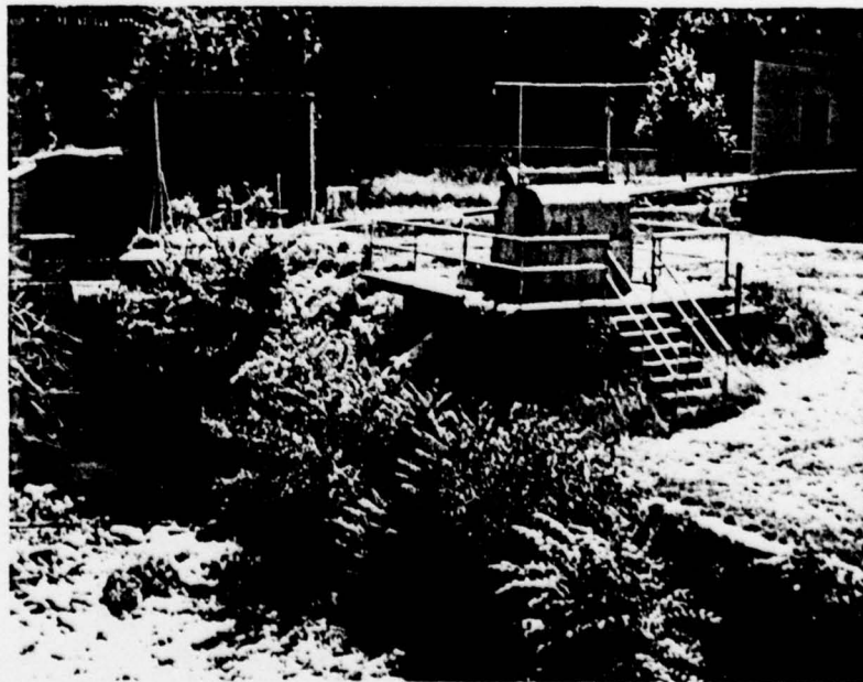
View of intake structure
