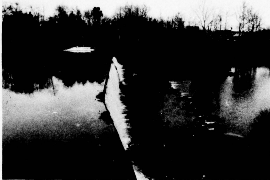
Photo 5 View along spillway crest looking towards left abutment
