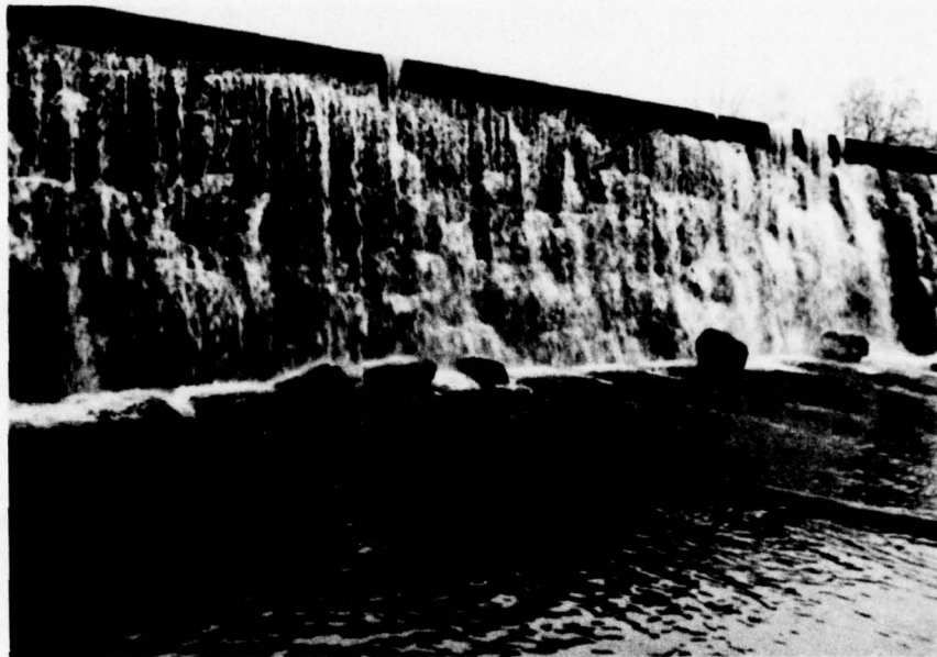
Photo 7 View of spillway face showing loose stones on apron
