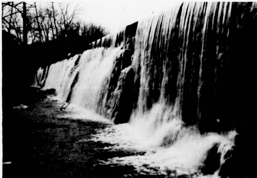
Photo 6 View of spillway face looking west from left abutment
