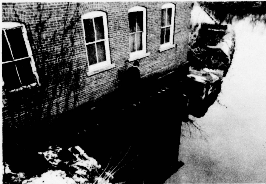
Photo 3 View of mill at right abutment of dam looking east
