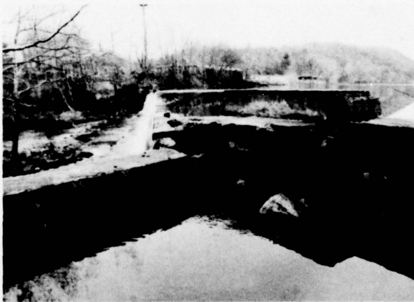
Photo 2 View of left spillway abutment looking west
