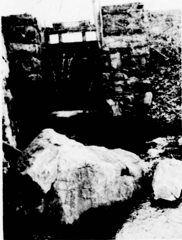
Photo 9 View of sluice gate looking upstream
