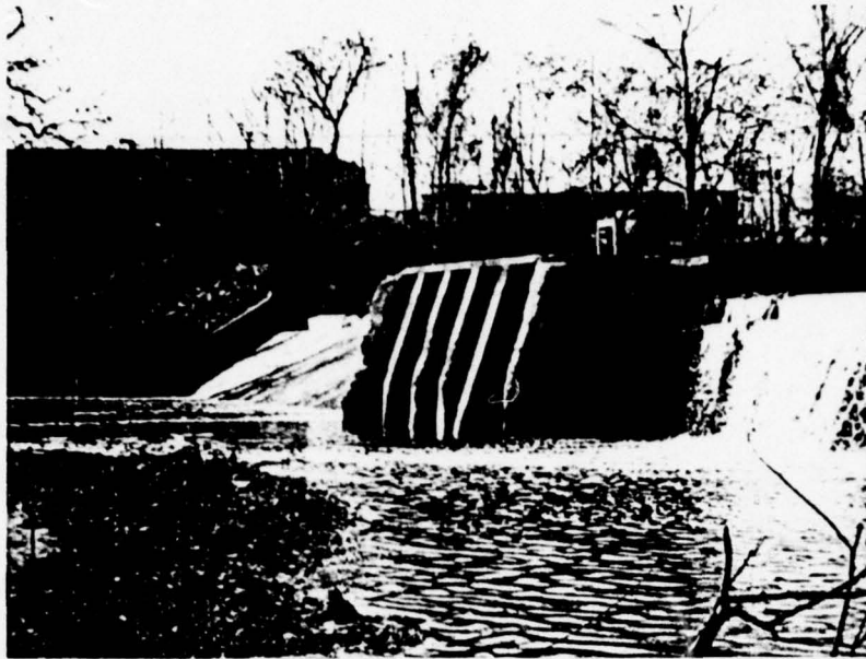
View of floodgate structure
