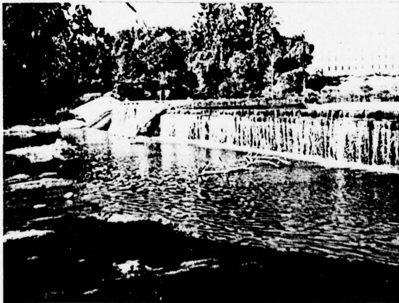
Downstream view of dam
