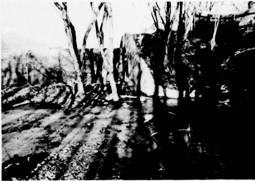
Photo 3 View of left abutment looking upstream
