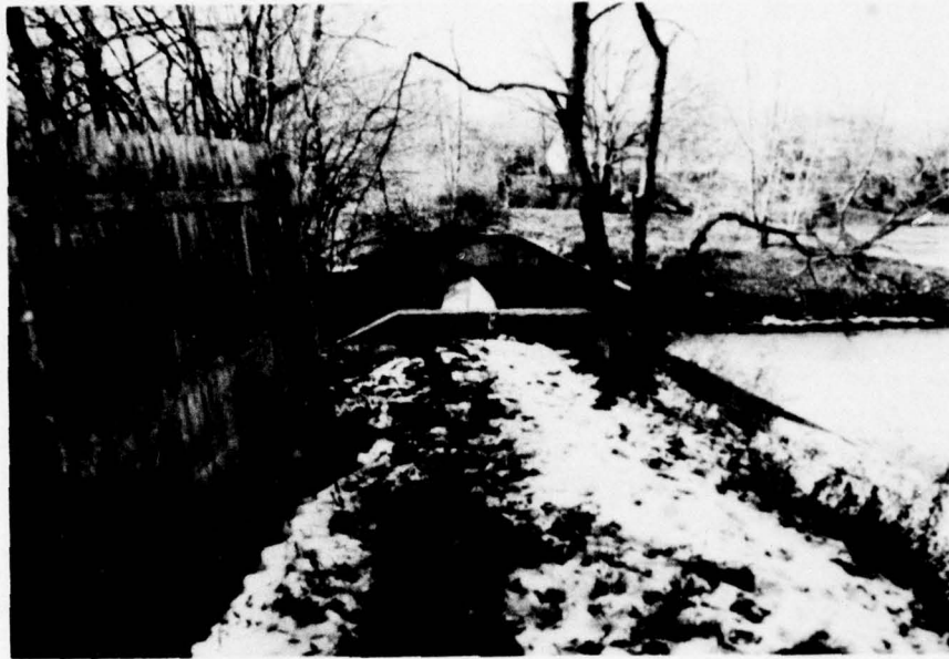
Photo 1 View along dam crest looking west
