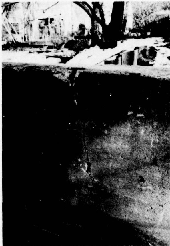
Photo 7 View showing crack in left (east) wing wall
