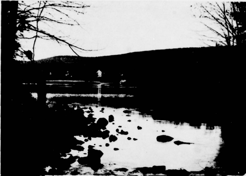
Entrance to Spillway
