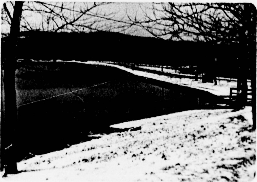
Photograph No. 2 Spillway approach. Spillway crest behind wood fence.
