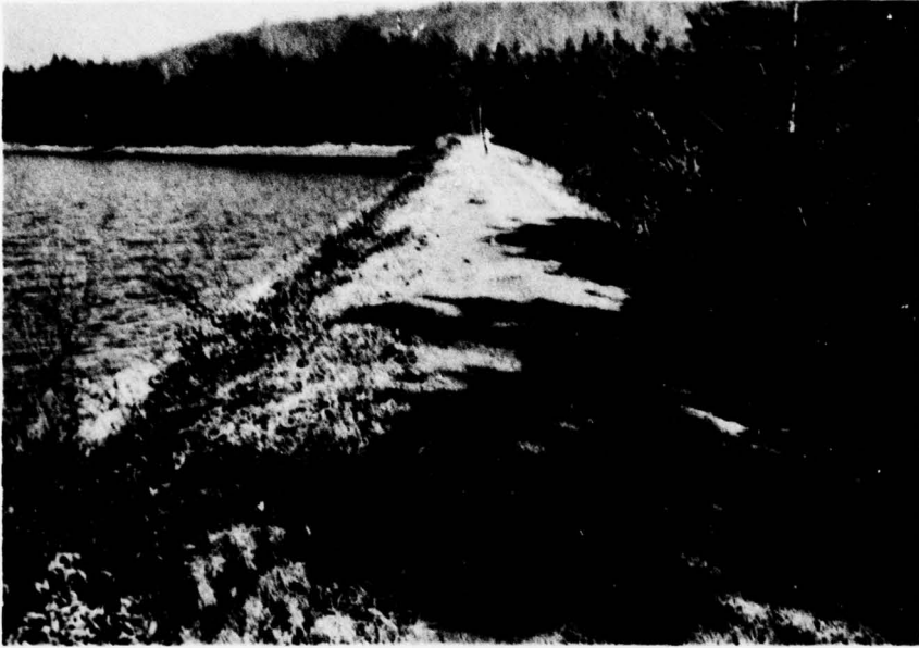
A. South Embankment - View from Right Abutment.
