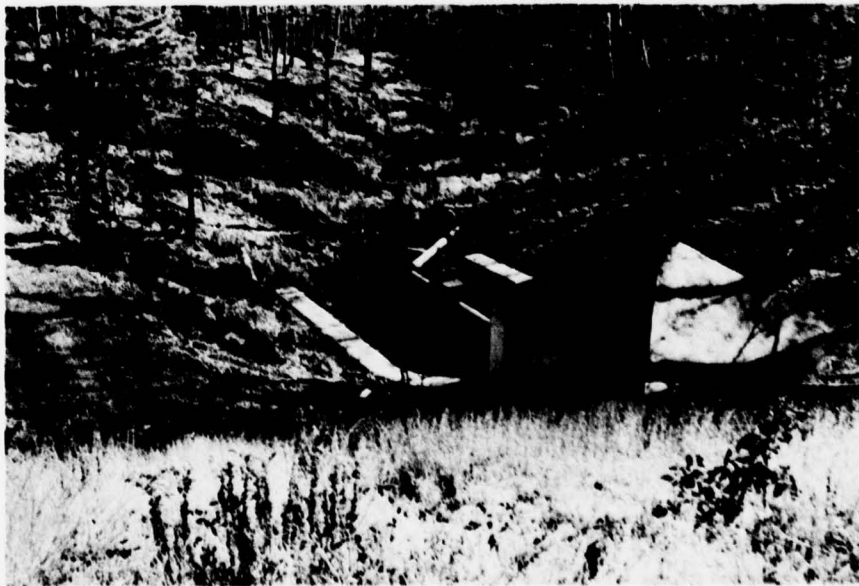
D. Downstream Channel.
