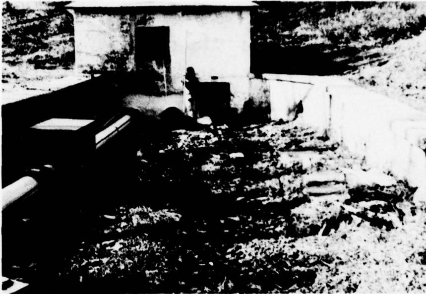
C. Spillway and Outlet Works Outlet
