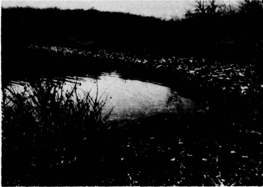
E. North Embankment - Upstream Slope.
