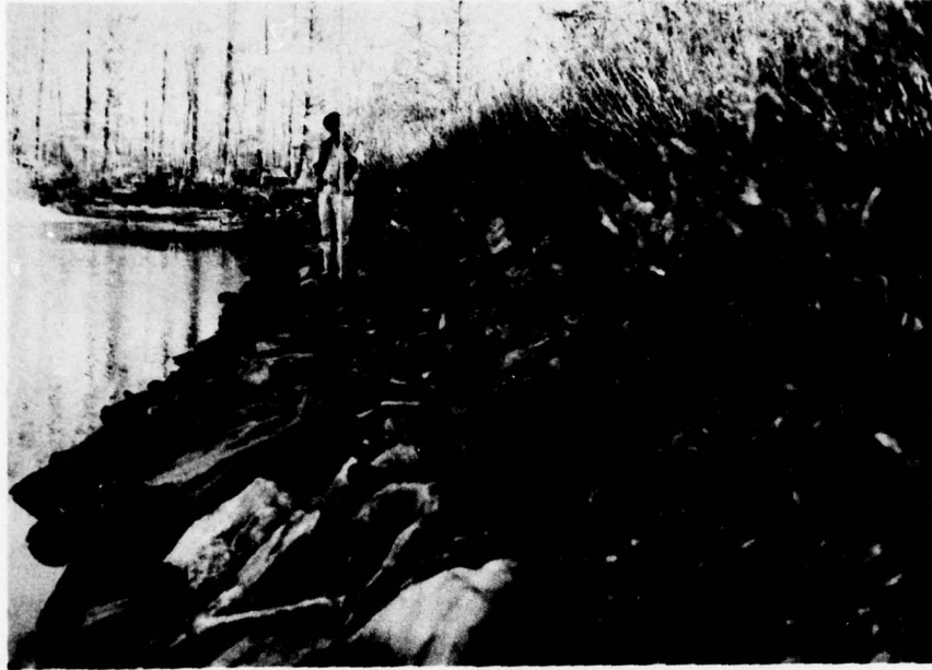
C. Upstream Slope of Embankment.
