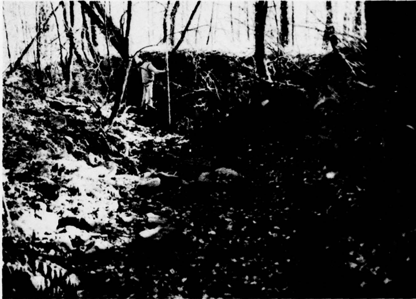
G. Spillway Outlet Channel - Looking Downstream.
