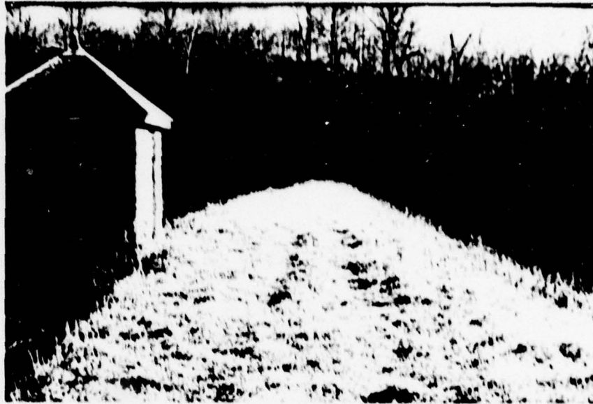
Photograph No. 1 Crest (looking east).
