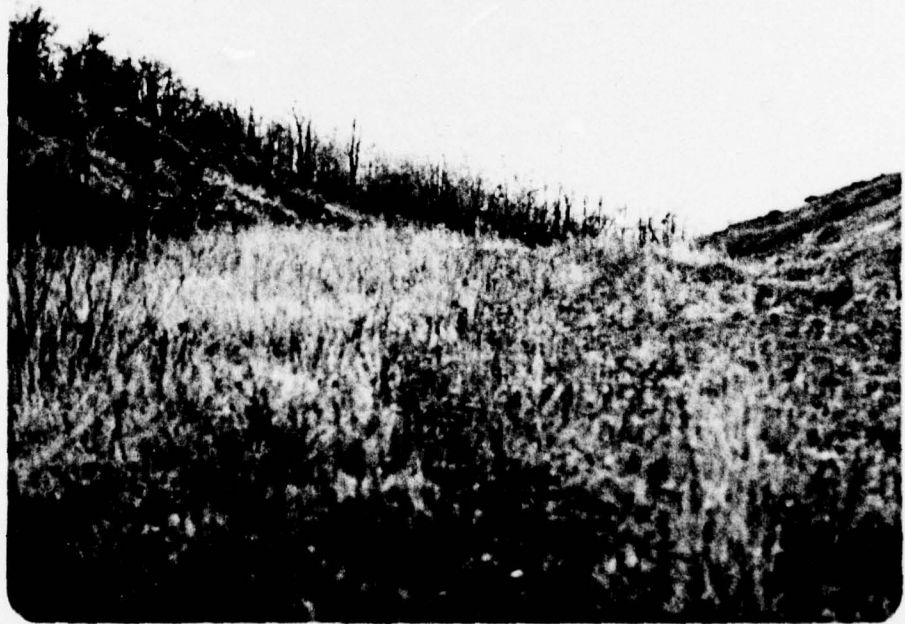
Photograph No. 2 Emergency spillway discharge channel.
