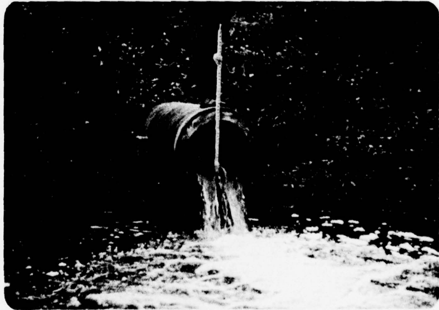
Photograph No. 4 Outlet pipe.
