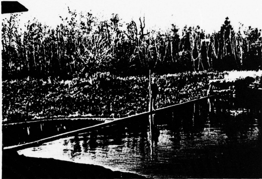
E. Spillway Approach Channel
