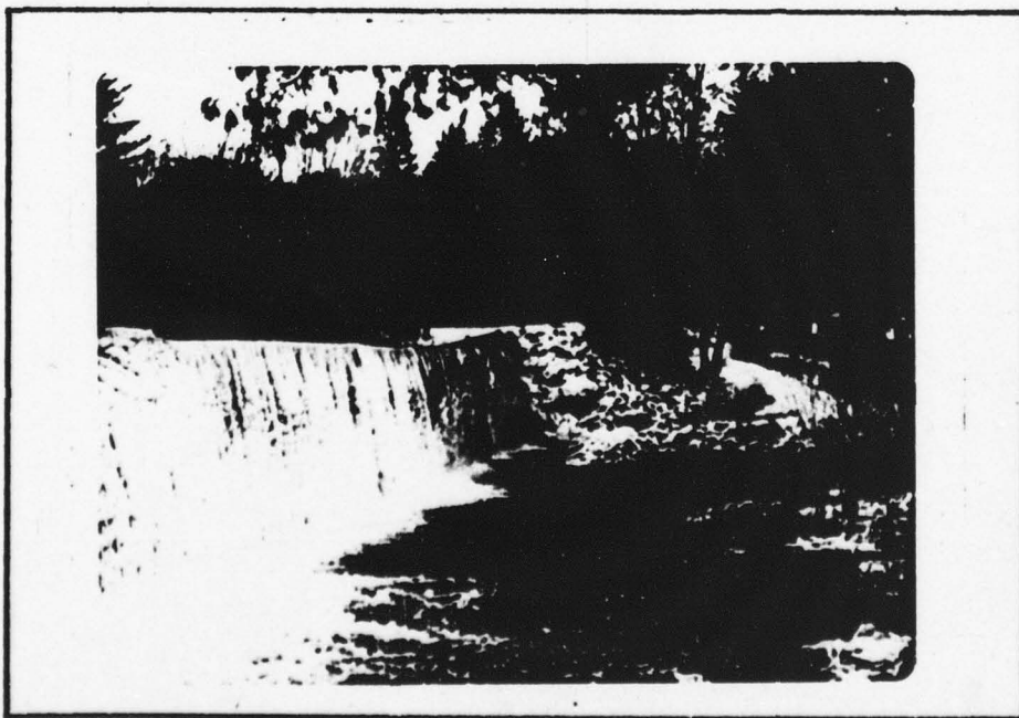
DOWNSTREAM VIEW OF THE DAM
