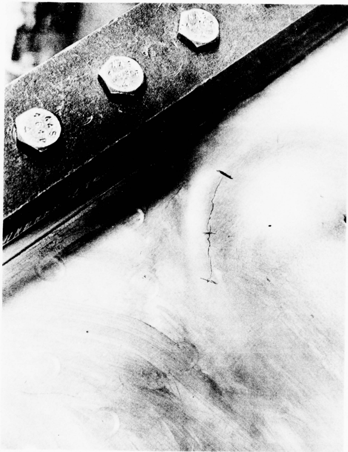
FIGURE 12. WELDBONDED PANEL FATIGUE CRACK AT 22,180 LOADING CYCLES, BEAD B
