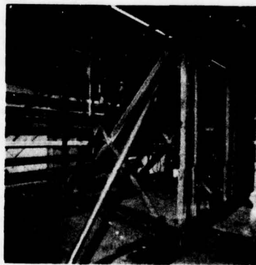
Figure A4. Interior of sled building before application of plywood skin.
