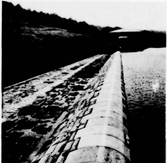
VIEW OF SPILLWAY
