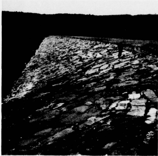
UPSTREAM FACE OF DAM
