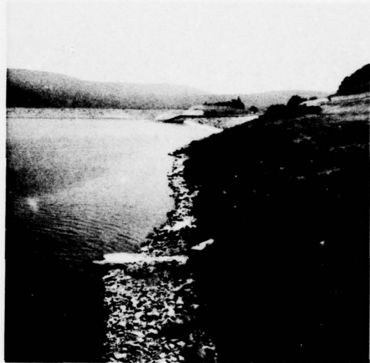
UPSTREAM FACE OF DAM, SPILLWAY AND RIGHT BANK OF RESERVOIR
