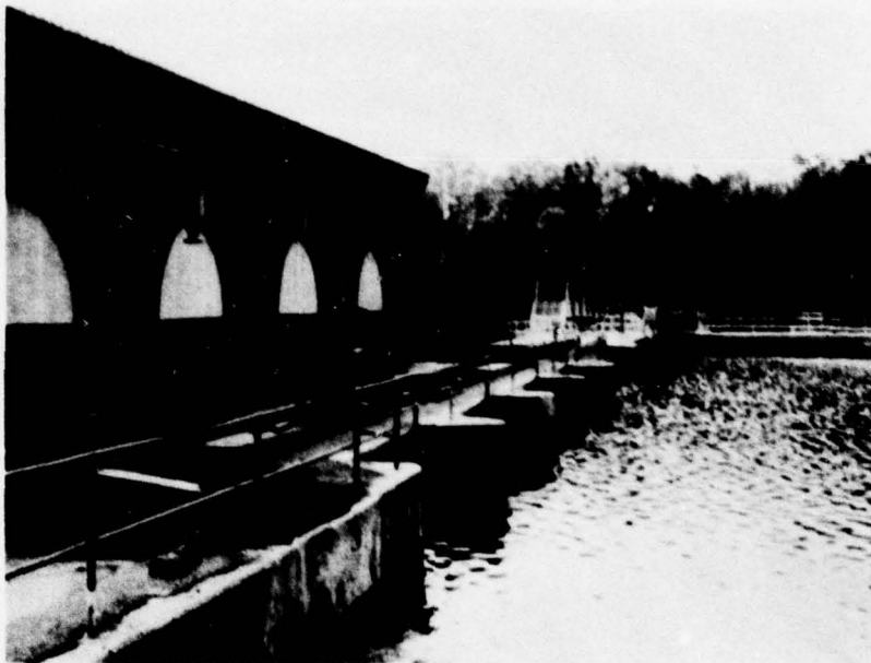
UPSTREAM FACE OF DAM FROM NORTH EMBANKMENT
