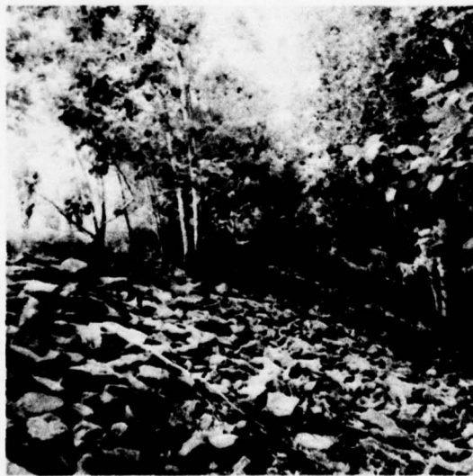
DOWNSTREAM FACE OF WEST DIKE
