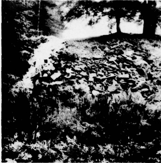
CHANNEL DOWNSTREAM OF SPILLWAY
