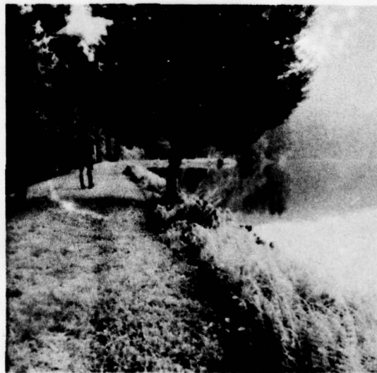
OVERALL VIEW OF WEST DIKE
