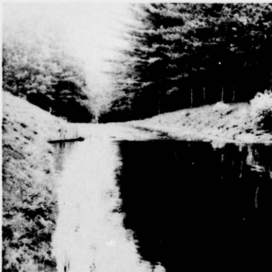
○ VIEW UPSTREAM AND DOWNSTREAM OF SPILLWAY
