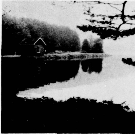
OVERALL VIEW OF COOPER LAKE DAM
