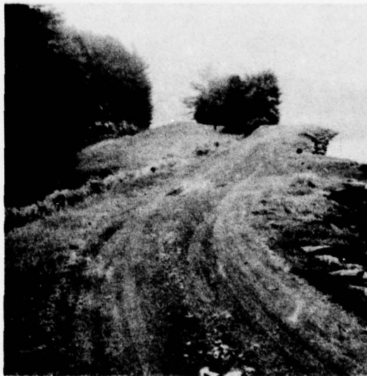
VIEW OF TOP OF DAM
