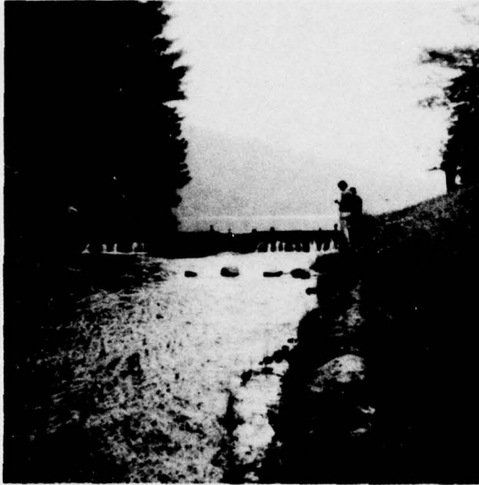
CHANNEL DOWNSTREAM OF SPILLWAY
