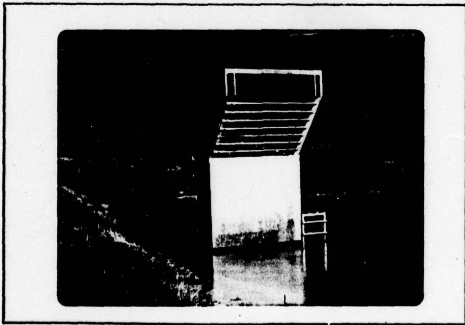
RISER SHOWING DETAILS OF BOTH THE HIGH STAGE AND LOW STAGE INLETS
