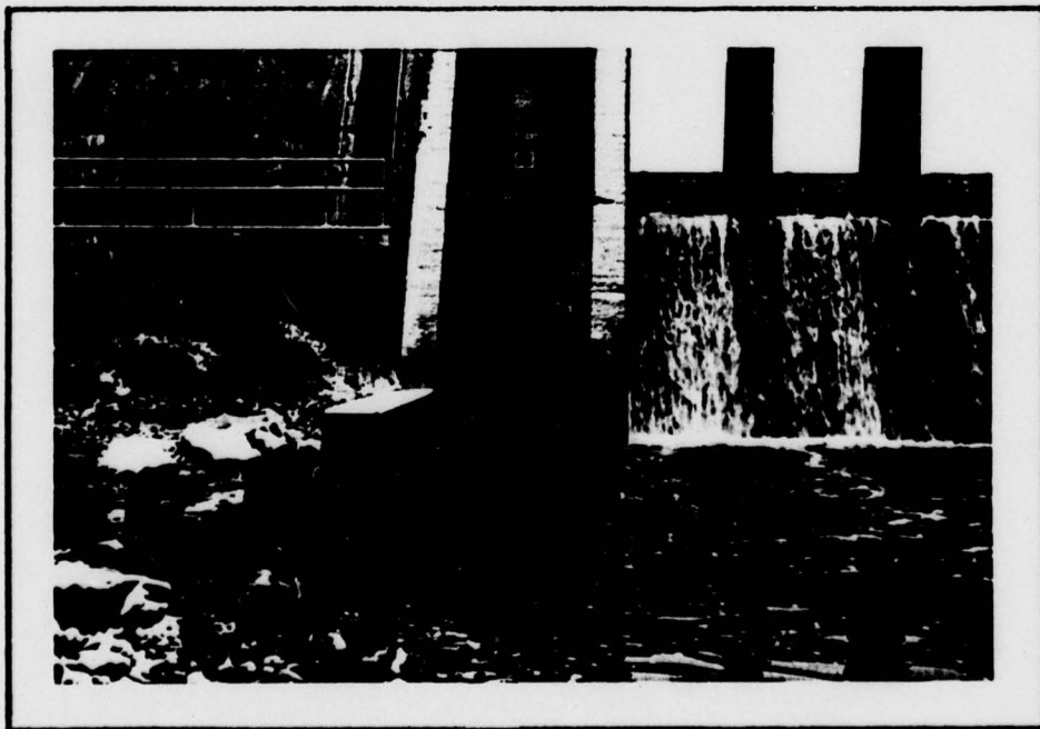
RESERVOIR DRAIN AND STOP LOGGED PORTION OF SERVICE SPILLWAY
