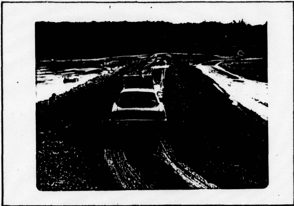
VIEW LOOKING ACROSS THE TOP OF THE DAM FROM THE RIGHT ABUTMENT
