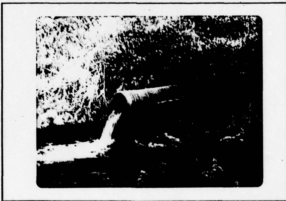
CLOSE UP OF THE PRINCIPAL SPILLWAY OUTLET SHOWING A DRAINAGE SYSTEM OUTLET PIPE
