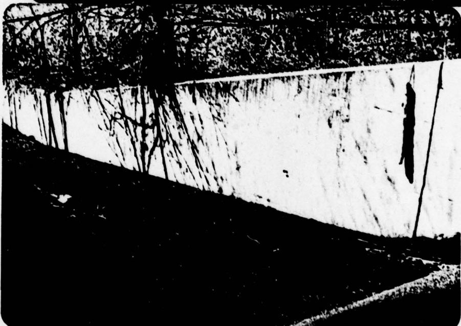
Right Wall Spillway Chute
