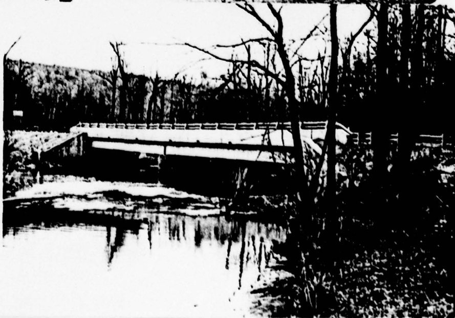
Two Span Bridge Downstream Channel
