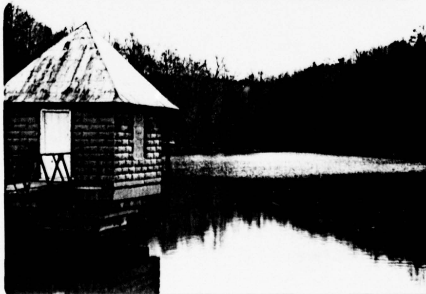
Reservoir and Control Tower
