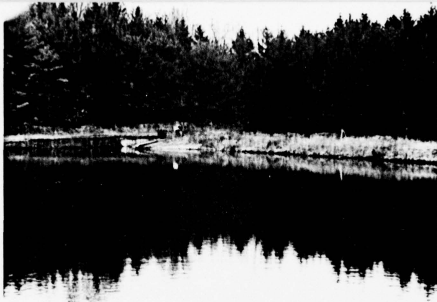
Upstream Slope and Forebay
