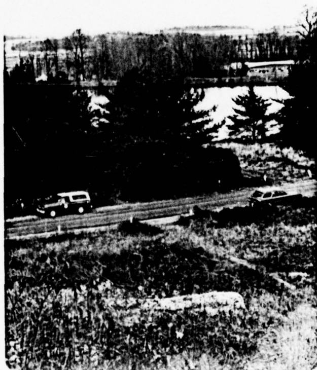
Looking From Dam To Downstream Reservoir
