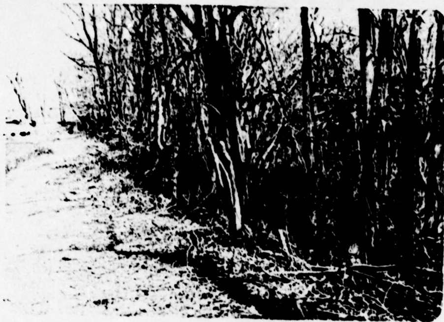
Dam Crest and Downstream Slope
