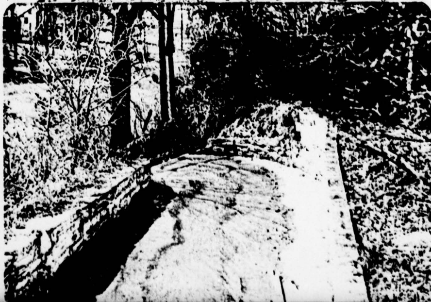
Top of Spillway Chute
