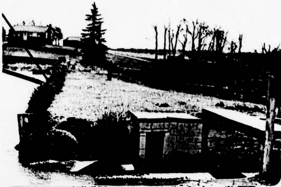
"Duck House" at Spillway Bridge
