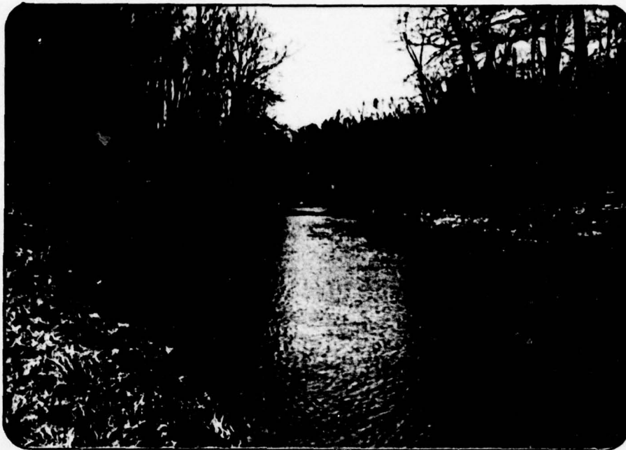
PHOTO 5. Downstream Channel as seen from Emergency Spillway Exit
