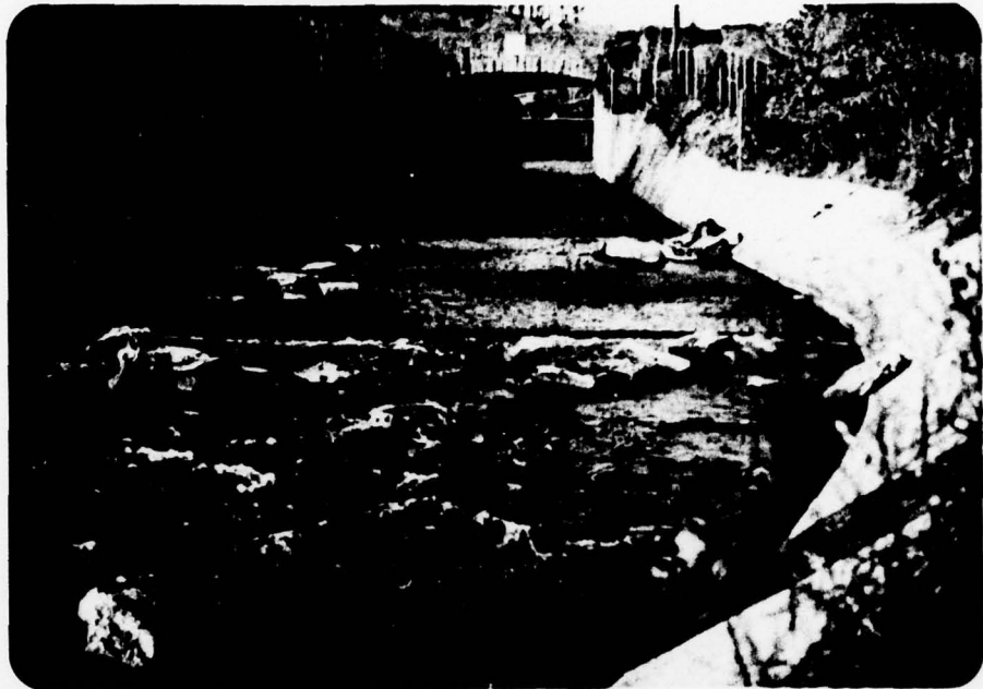
Photograph No. 3 Spillway discharge channel.
