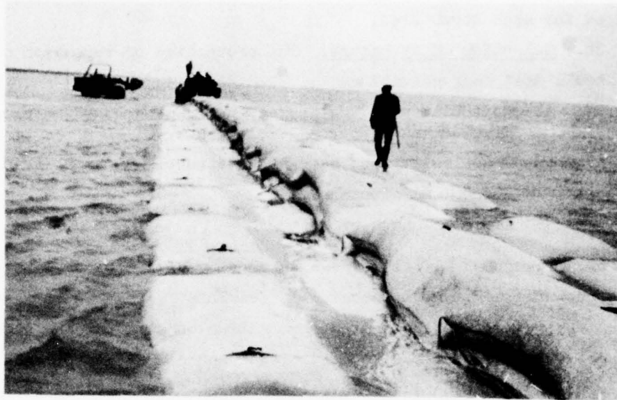
a. Dike construction
