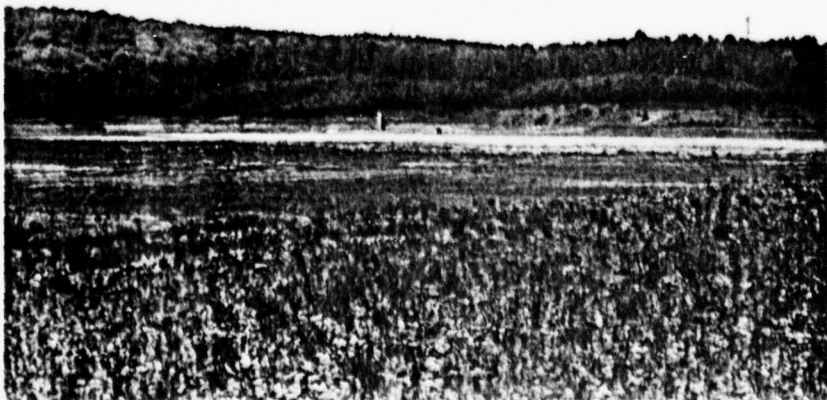
View from top of dam towards decant towers
