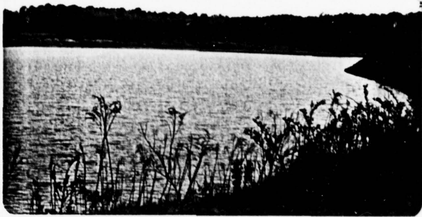
Reservoir - Dam in background
