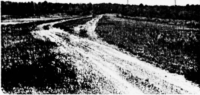
Top of Dam Looking to Left Abutment
