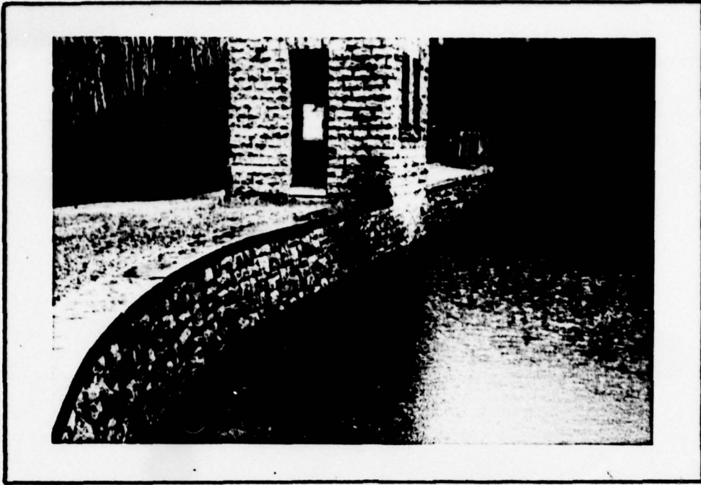
UPSTREAM FACE OF THE DAM SHOWING THE GATE HOUSE AND THE VEGETATION GROWING FROM THE MASONRY WALL
