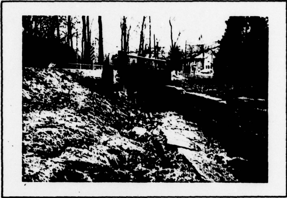
SPILLWAY OUTLET CHANNEL LOOKING DOWNSTREAM TOWARDS THE BRIDGE SECTION WHICH IS ABOUT 400 FEET DOWNSTREAM OF THE DAM
