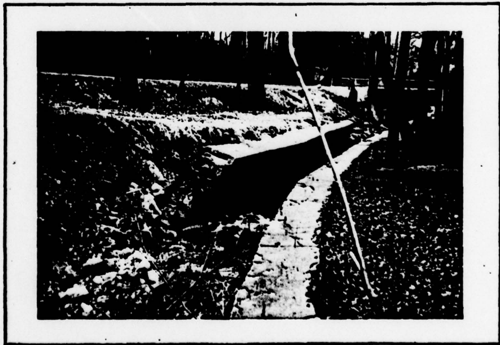
LOOKING DOWNSTREAM AT THE CRUMBLED AND DISPLACED LEFT TRAINING WALL IN THE SPILLWAY OUTLET CHANNEL
