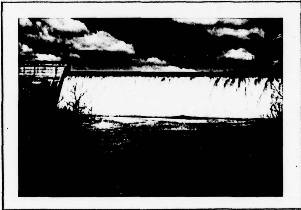
LOOKING UPSTREAM AT THE OVERFLOW SPILLWAY
