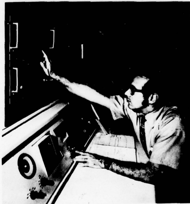
Linear Accelerator Control Console
