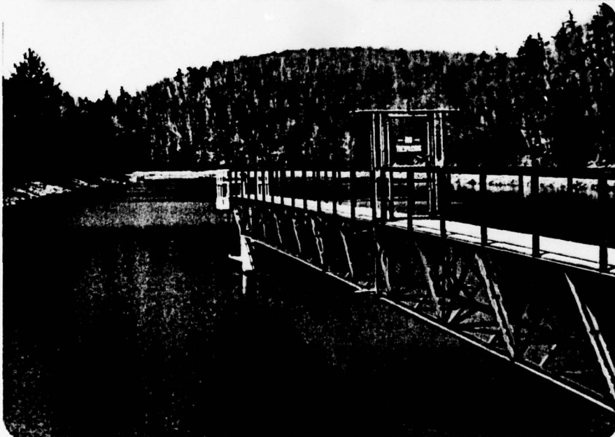
Bridge to intake Structure.
