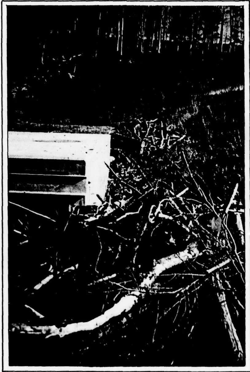
TRASH REMOVED FROM INTAKE RISER AND PILED AROUND STRUCTURE.
